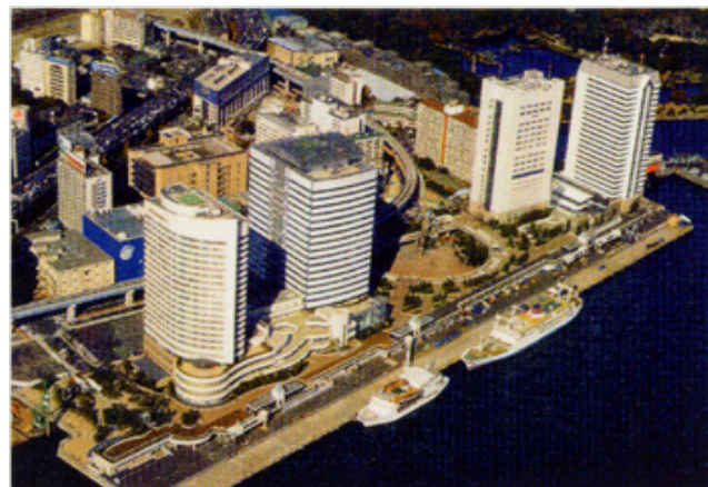
Takeshiba Wharf Improvement Project
